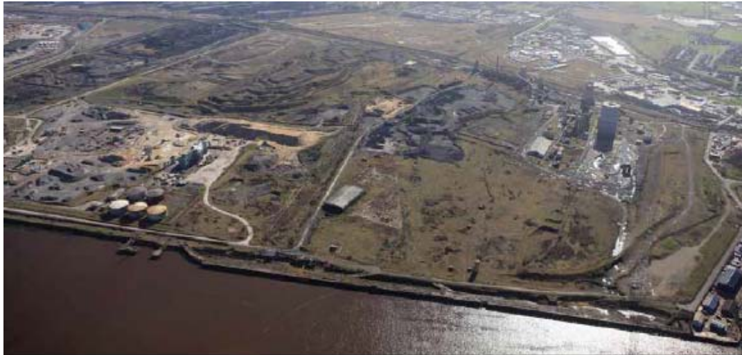
Figure 2.1 Aerial view of application site
